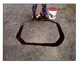
preferably moist or damp. If necessary, dirt, loose pieces of asphalt or concrete material, and excess water in the saw cut shall be removed with an air jet. The surface of the surrounding pavement should be air-dry when the application of OverKote Loop Filler is made. OverKote Loop Filler should be thoroughly stirred before use, and protected from freezing. OverKote Loop Filler should be used as received
