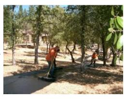
should be avoided. Sealcoat should be completely dry before a second coat is applied. The sealcoat should be fully cured before allowing traffic to drive on it or markings to be applied. A good sealcoat job performed by a qualified contractor should last between 2 and 5 years.
