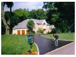
provided here. First, all debris and dirt needs to be removed from the area to be sealcoated. This can be achieved with wire brooms, blowers, vacuums, sweepers and/or pressure washers. Second, all potholes, cracks and depressions need to be filled. Third, any areas of thick paint from markings may need to be ground off. Finally, all contaminated areas of asphalt need to be treated.
